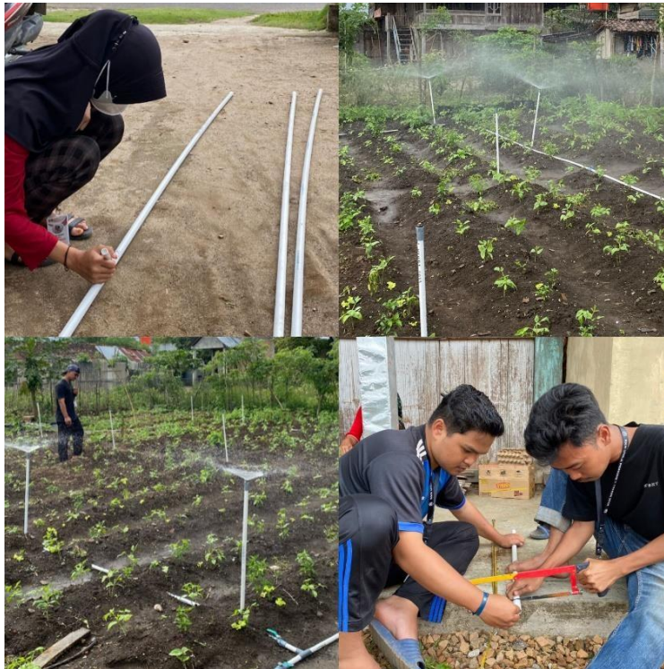
Gambar 1. Proses Instalasi Sprinkler
